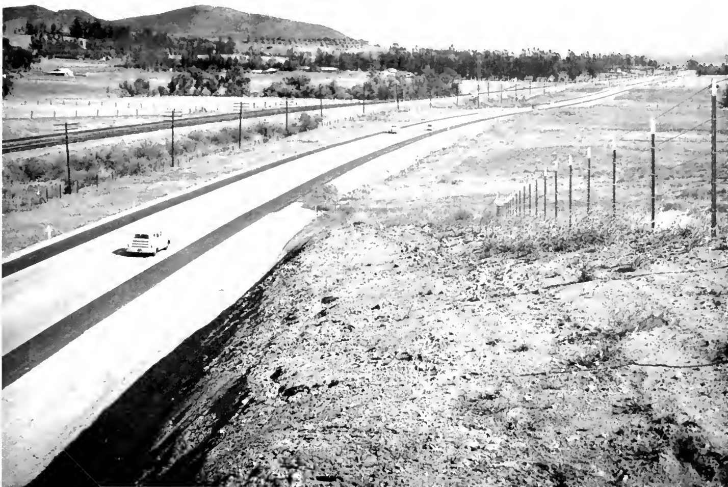
Typical alignment of Arlington-Mira Loma Expressway recently completed by Riverside County under the Federal Aid Secondary Highway Program
